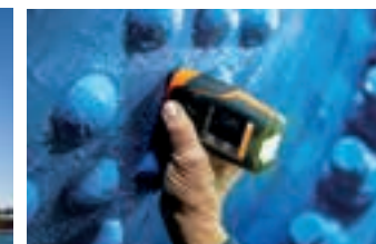
Limit monitoring via light
